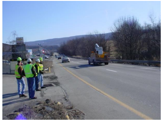
Figure 11 SR-119 Looking North
