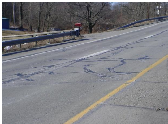
Figure 13 Fatigue Cracking
