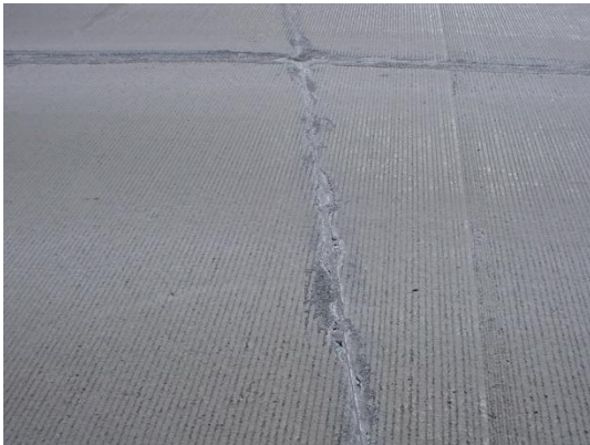
Figure 20 Freeze-Thaw Deterioration
