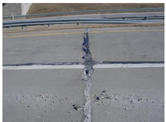
Figure 25 Freeze-Thaw Deterioration
