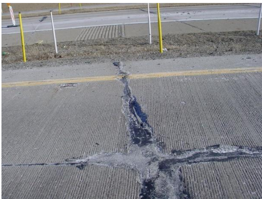
Figure 24 Freeze-Thaw Deterioration
